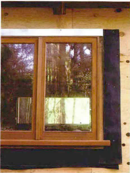
Flashing and blind stops. Once the window and the tar-paper splines are in place, blind stops the same thickness as the boards are nailed around the sides and the bottom of the window. The head flashing extends to the edges of the side blind stops (above) and is covered with the top layer of tar paper, a blind stop and the head casing (below).
