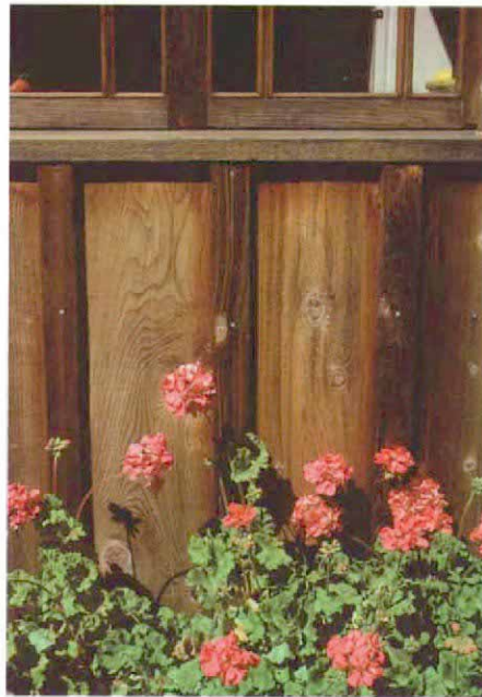
Left to weather. Unfinished and rough-sawn redwood boards cover the author's house.
