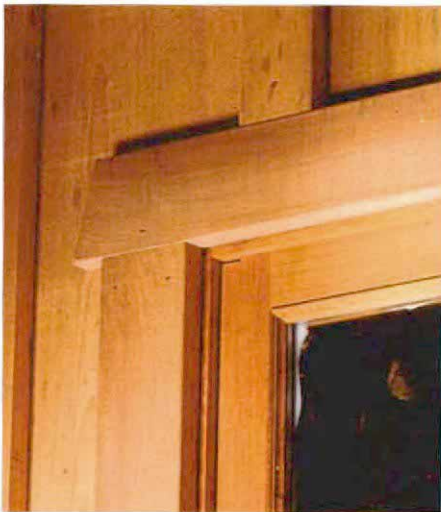
Flashing and blind stops. Once the window and the tar-paper splines are in place, blind stops the same thickness as the boards are nailed around the sides and the bottom of the window. The head flashing extends to the edges of the side blind stops (above) and is covered with the top layer of tar paper, a blind stop and the head casing (below).
